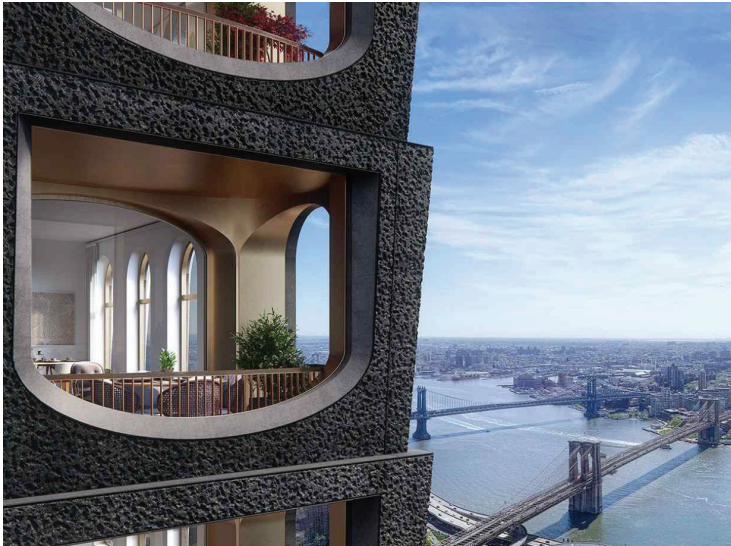
At 130 William, Sir David Adjaye designed a hand-cast concrete façade to create a striking form against the cityscape of Lower Manhattan
